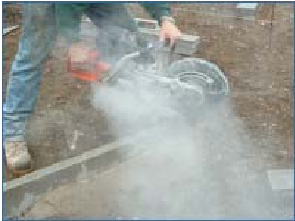
3. Kerb cutting prior to laying
