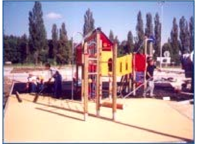
16. Kerbstone perimeter installed
