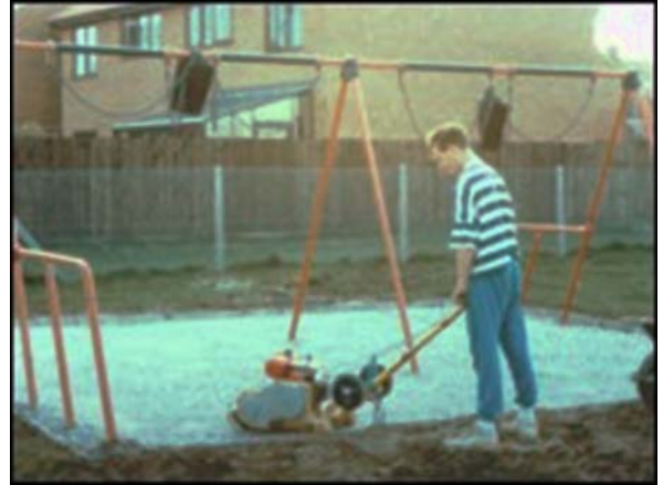
8. Levelling stone foundation
