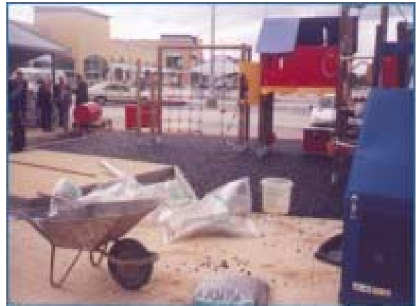
10. Laying base rubber
