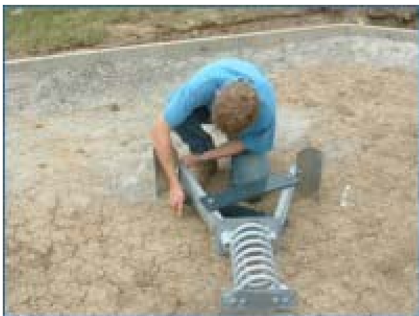
5. Installing play equipment
