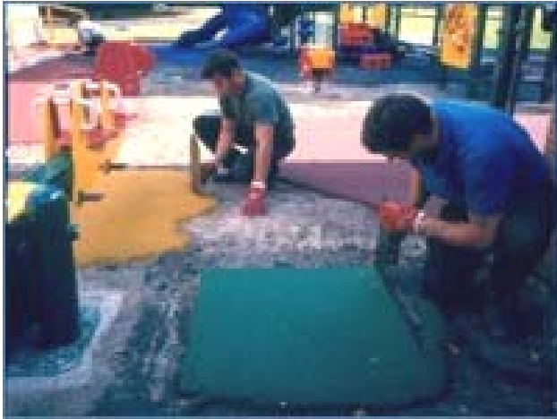
15. Kerb cutting prior to laying
