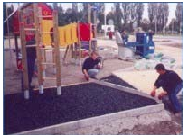
12. Levelling base rubber
