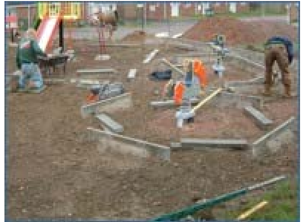
4. Kerbstone perimeter installed
